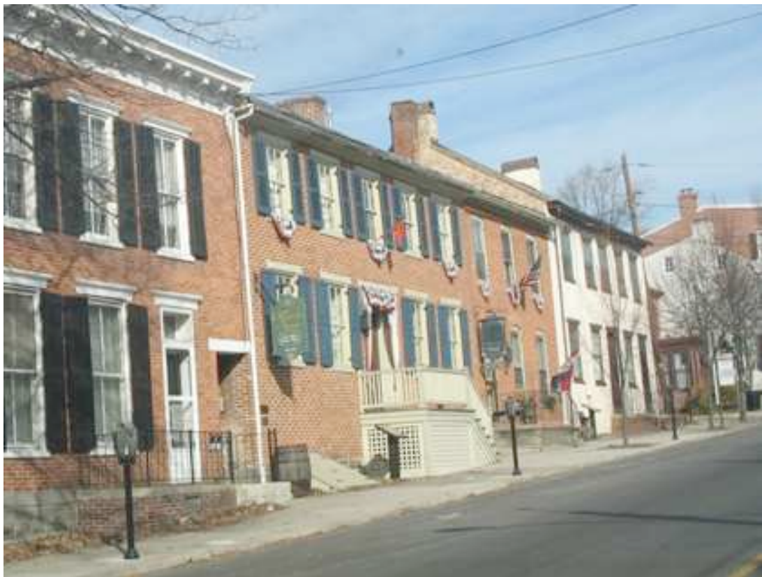
Figure 1. Shriver House on Baltimore Street in Gettysburg, Pennsylvania.
